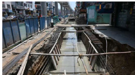
Tardy progress A stormwater drain being built on Kallamman Road at Vinugambakkam. Residents are worried whether the remaining stormwater drain work will be completed in time. B. VELANJANANI (RA)
